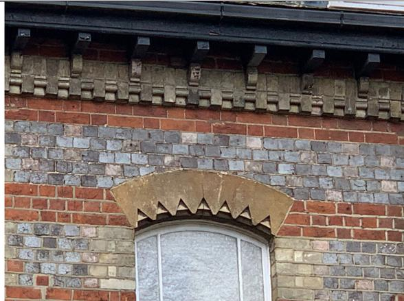
Fig 5.: Architectural Details - Villa entry porch to front door. Decorative banded brickwork.
